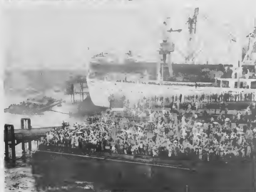
A LARGE crowd witnessed the event. Launching a ship the size of the new Esso Aruba requires considerable forethought and is attended by some risk. The vessel must be stopped quickly either with its anchor or strong cables from the bow attached to heavy piles of chain. UN GRUPO grandi a mira e evento. Bahamento na awa di un bapor di tamanjo di Esso Aruba ta requeri considerable planeamento y ta bay acompaña di algun riesgo. E tanquero mester wade para liberamente sea cu su ancla di cablenan fuerte mara.
